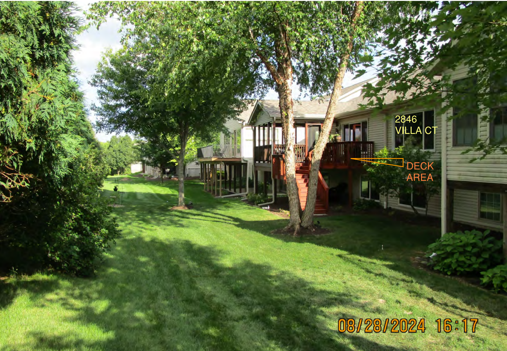
2846 DECK BUILD OUT LOCATION
